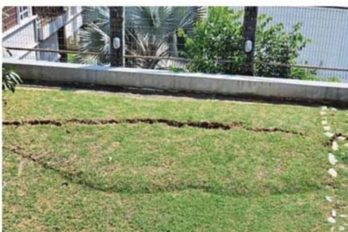
Tension cracks indicate ground movement and possible slope failure.
