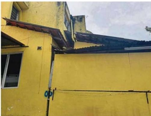
When the structures of a house move from their original position, this can be a sign of slope development failure.
