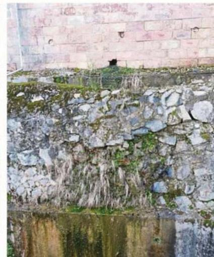
A bulging wall due to water pressure at the base of a slope or retaining wall.
